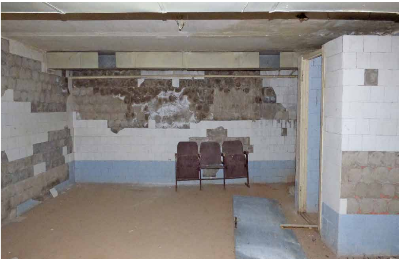
Basement of the former Kindrashivska-Nova ambulance station building
